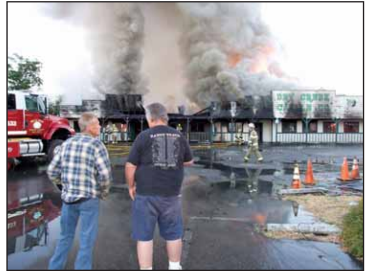
Jeff Miller (right) owner of Dry Creek Station and employee Stan Friberg watch the fire move through the attic from the lounge to the dining room of the restaurant. Firefighters were unable to gain access to the flames from below due to the one-inch tongue and groove ceiling above the beams.
